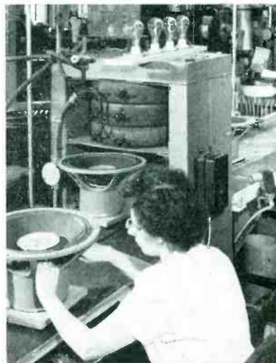
Assembly line for high-fidelity loudspeakers, with 2½-ton magnetizer straddling conveyor belt that runs over top of bench. Light beam goes diagonally through magnetizer from right front of bench to phototube at left rear. Surge-absorbing lamps are on top of magnetizer frame.
