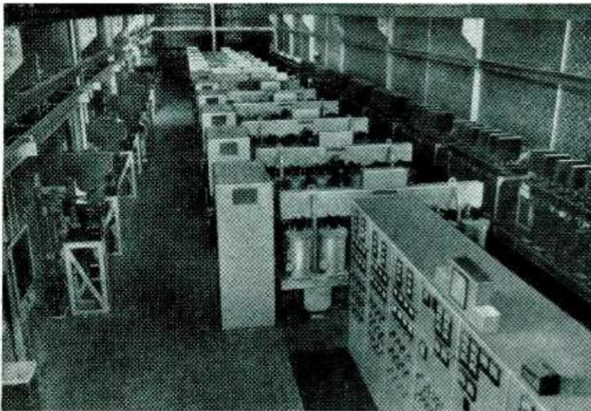
Rectifier station for an aluminum pot line. Anode and cathode circuit breakers are on right and left walls respectively. Master switchboard is in foreground
