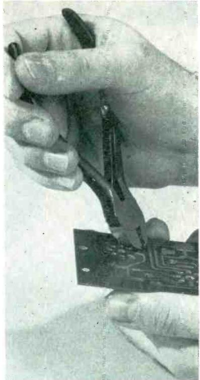
Method of holding new pliers to get optimum visibility while cutting and crimping leads. Replaceable tempered-steel springs keep pliers open, ready for immediate use
