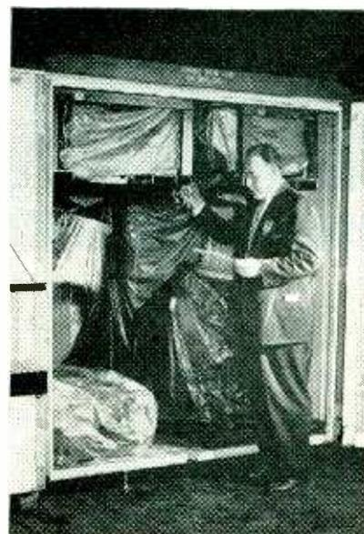
Appearance of Transportainer after all parts have been put in. When doors are closed and locked, equipment is protected just about as well as if in a safety-deposit vault. Parts are loaded in such a way that they can be removed in the correct numerical sequence for quick and easy assembly
