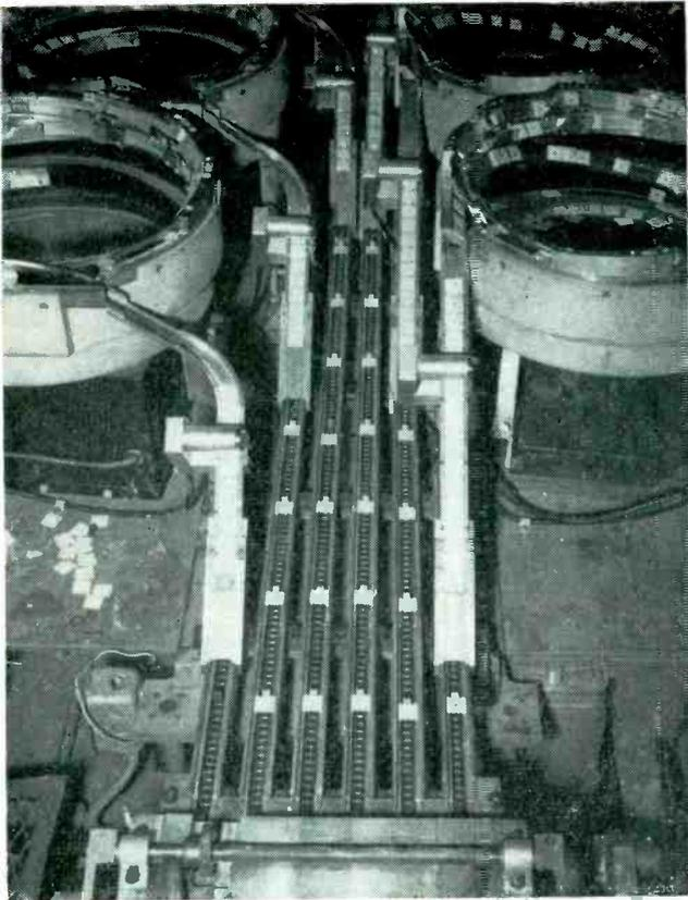
**PATTERN PAINTER** orients molded ceramic wafers and applies required pattern of silver paint to both sides of the six different wafers that are to make up a module. At left is input to machine.
