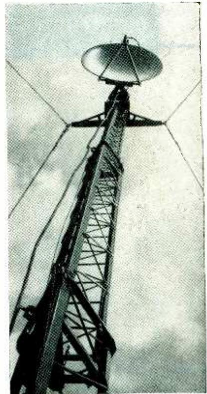
This 58-ft antenna mast telescopes to 20 feet for transporting
