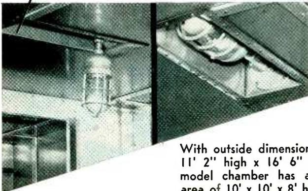
With outside dimensions of 13' 2" wide x 11' 2" high x 16' 6" long, this standard model chamber has an interior working area of 10' x 10' x 8' high. Door is 5' wide x 8' high, its window 30" x 30", and wall window 36" x 36".
