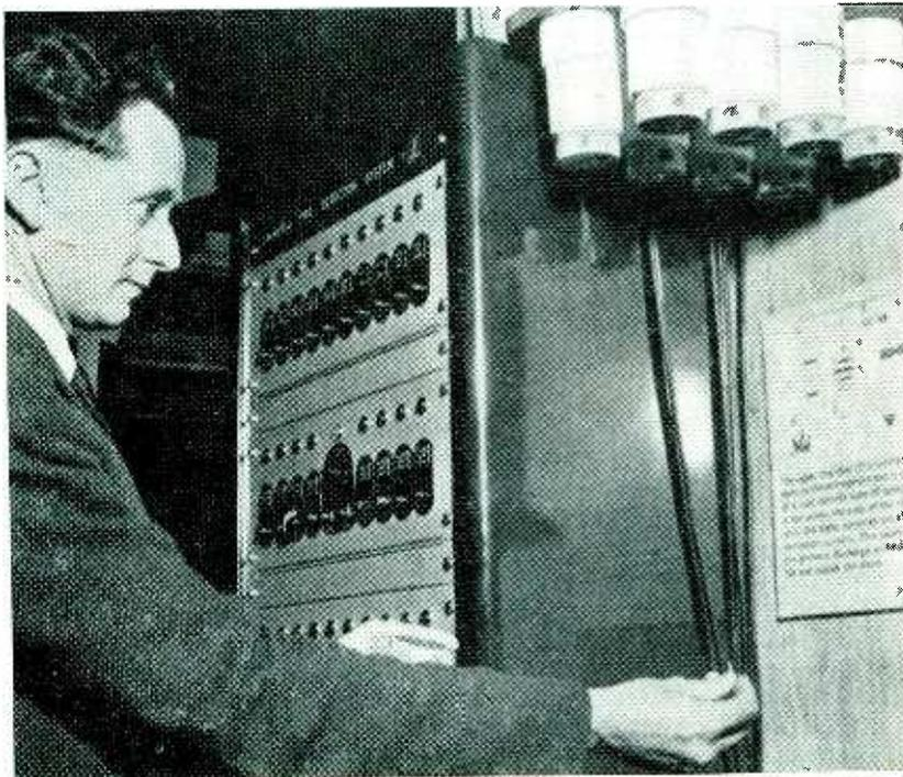
British device now in use by the Admiralty detects fires by means of small cells containing radioactive material. Each cell will protect from 20 to 50 yards of floor space. Its guaranteed life is 1,000 years. The least trace of smoke triggers an electrical bridge circuit containing a special cold-cathode tube that pulls in a relay to ring the alarm
