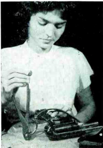
Method of using crimping tool to speed assembly of soldering gun
