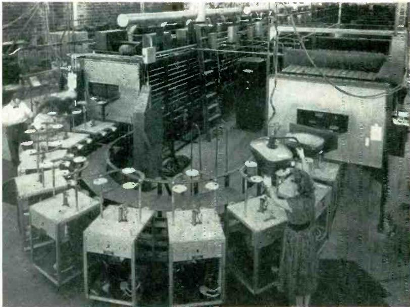
Loading and unloading end of picture-tube exhaust machine. Trolley wheels at top rear of each cart run on steel rail to guide caster-mounted carts on their 300-foot round trip through the U-shaped oven. Power trolleys on each cart pick up power for pumps and other cycling functions required during bake-out. Motorized conveyor chain keeps carts equally spaced as it moves them
